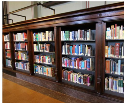
Fully adjustable, metal cantilever shelving was installed inside the original wooden cubbies where the damaged wooden shelves were removed.
